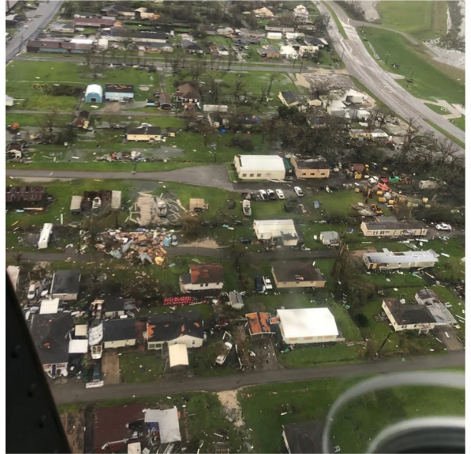
The U.S. Coast Guard conducted overflights Monday following the landfall Hurricane Ida. Aircrews conducted overflights near Galliano, LA to assess damages and identify hazards.
