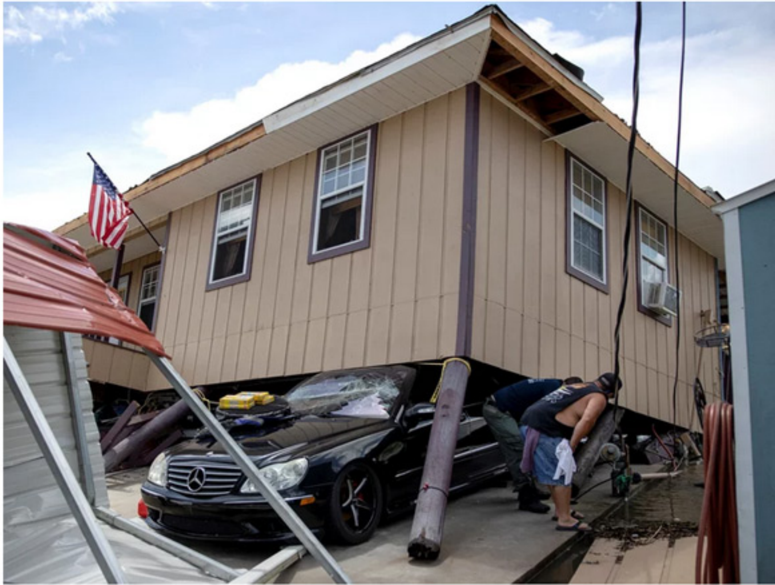
A man checks a broken gas pipe with a firefighter after Hurricane Ida hit Bourg, Louisiana, the United States, Aug. 30.
