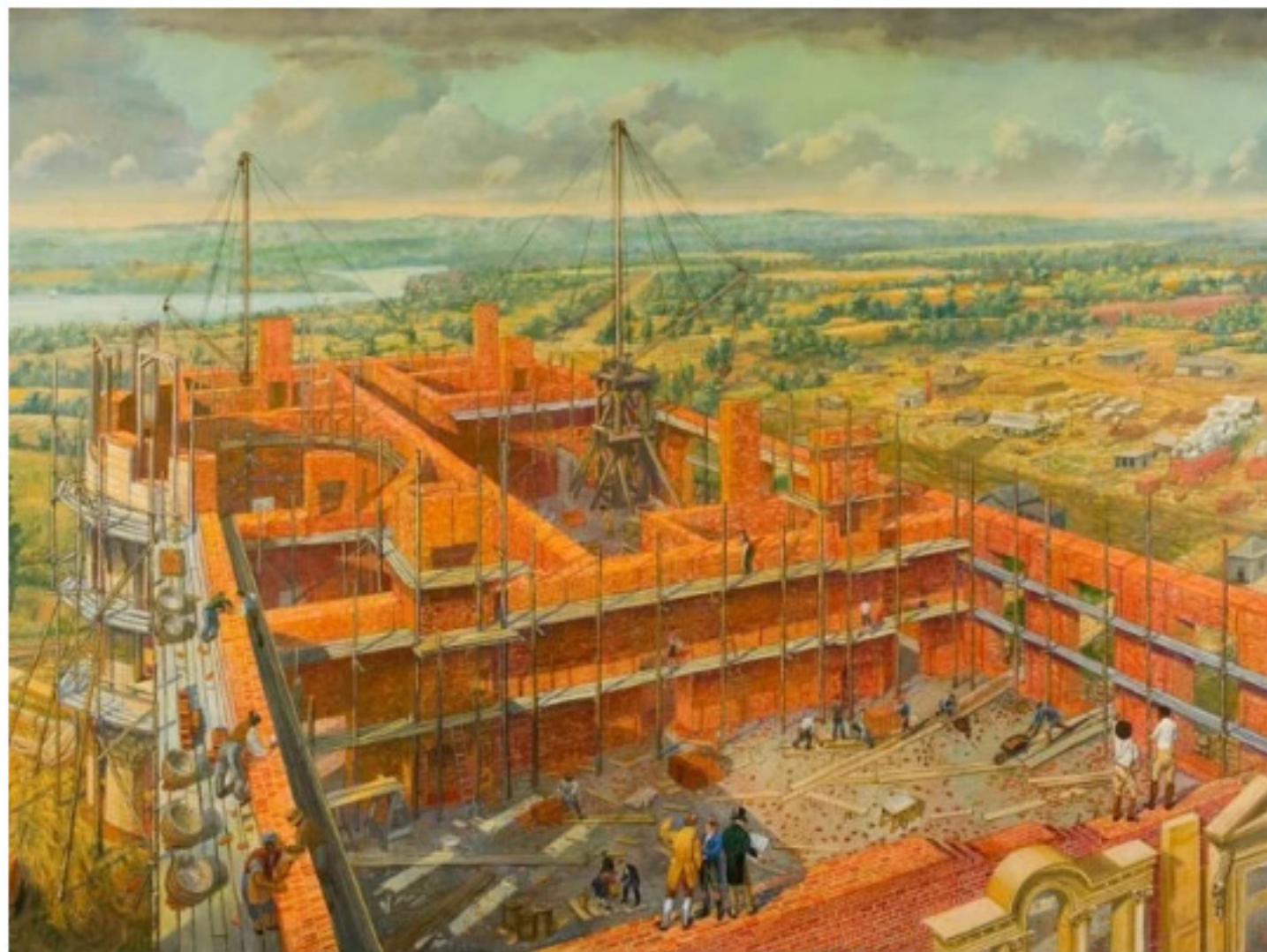
The WHHA commissioned this 2007 painting, "A Vision Takes Form" by Peter Waddell, to illustrate 18th-century construction of the White House as it may have appeared in 1796. The association is looking to find more information about the enslaved laborers who built the mansion.
