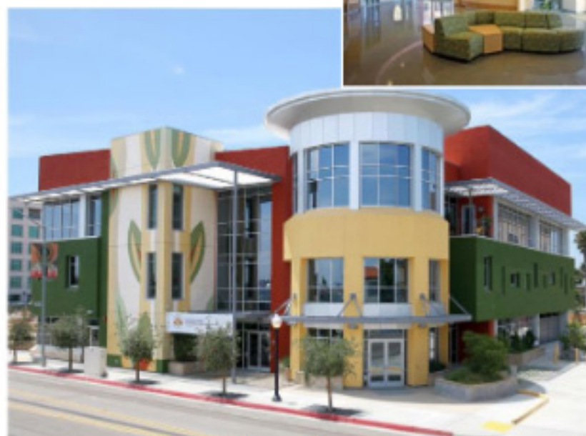
LEED Certified Gold Health Center, opened 2010
