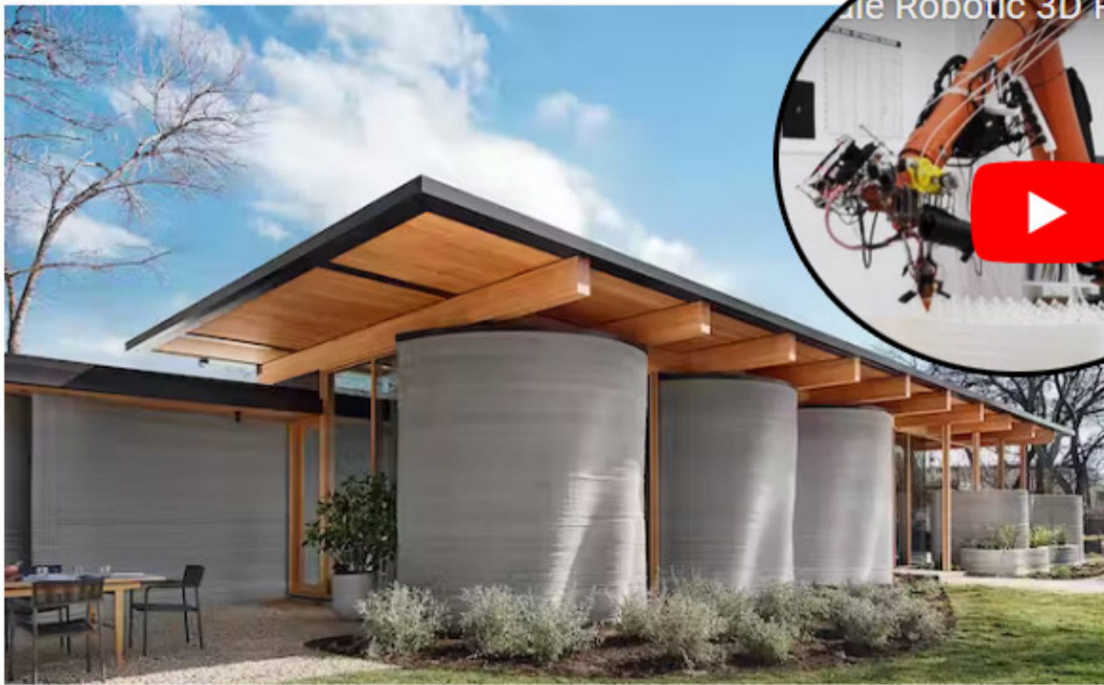
House Zero in Austin, Texas, is a 2,000-square-foot home that was built with 3D-printed concrete. Lake Flato Architects
