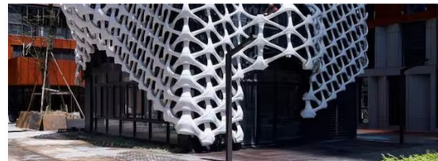
A 3D-printed façade in Foshan, China. The Association for Computer Aided Design in Architecture
