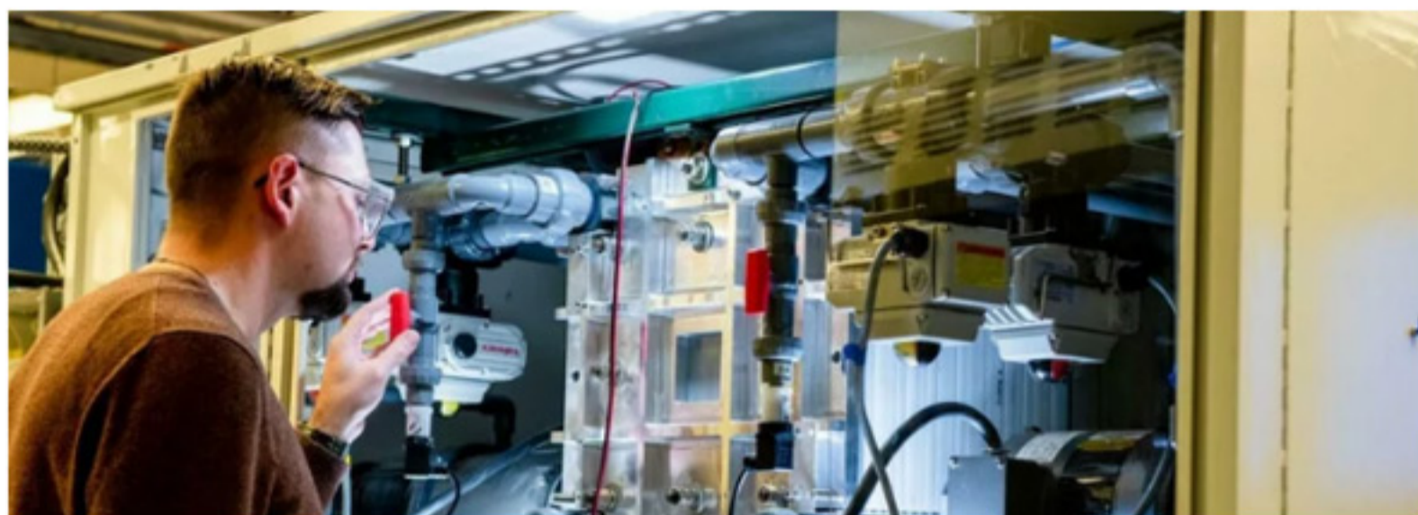
An employee examines a vanadium flow battery stack in the Battery Reliability Test Laboratory at PNNL.
