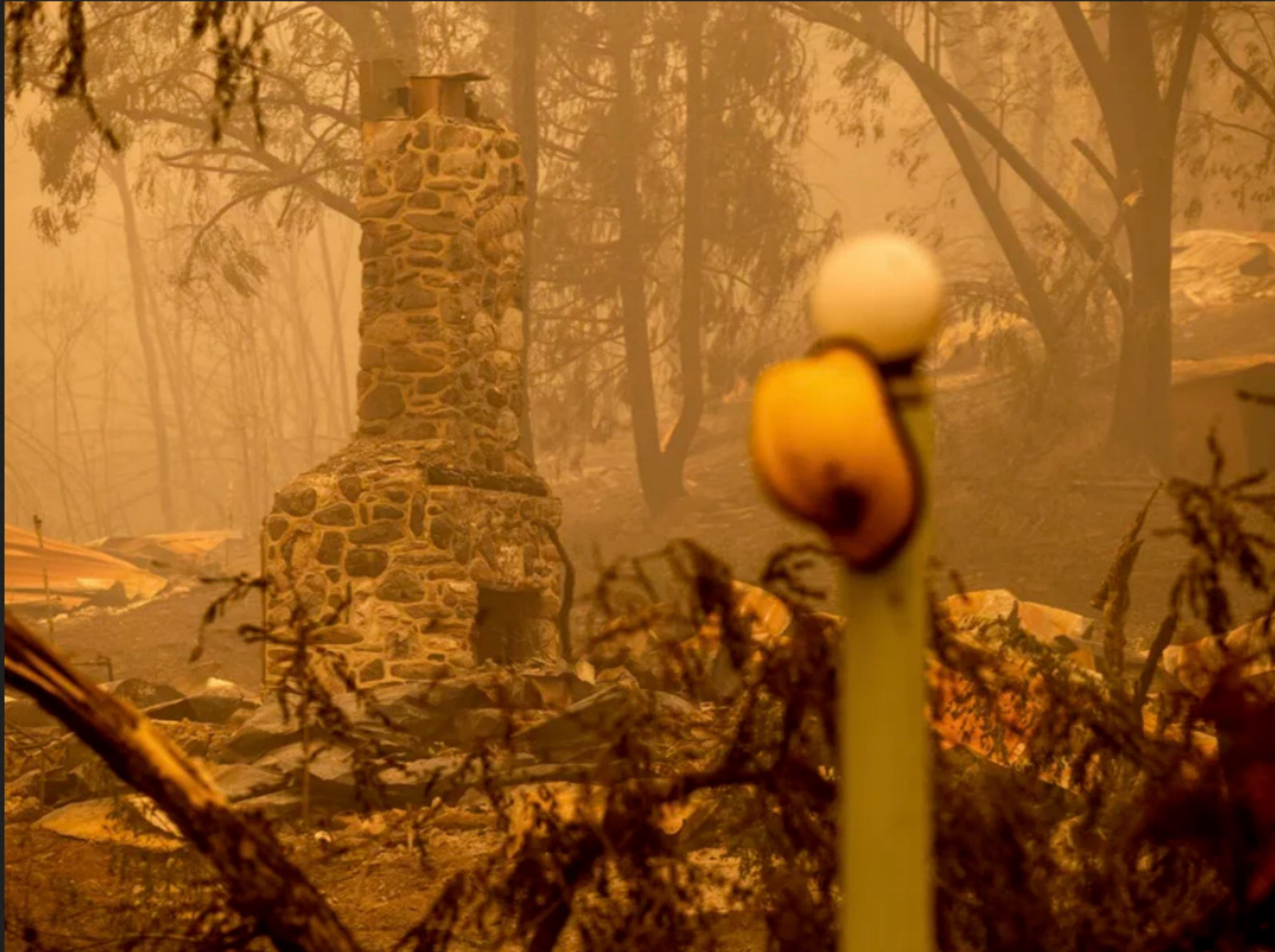
A chimney stands at a destroyed building as the McKinney Fire burns in Klamath National Forest, Calif., on Sunday.
