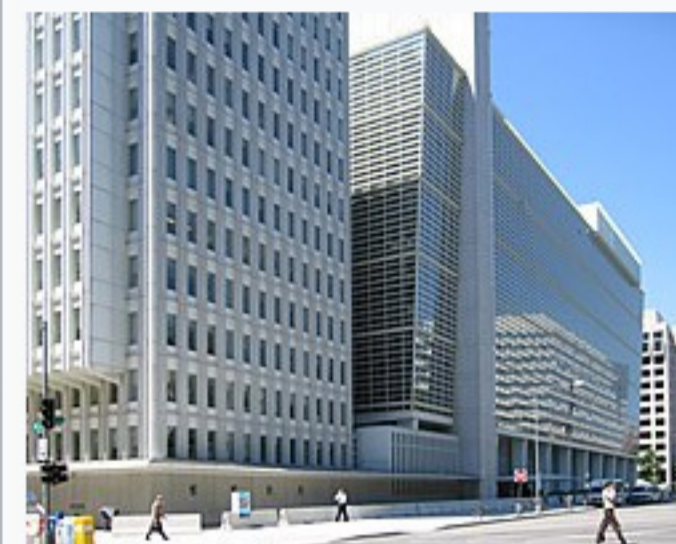
The World Bank Group building in Washington, D.C.
