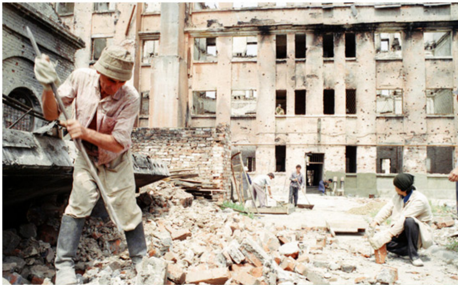
Residents of Grozny dig through rubble of destroyed buildings to salvage whole bricks to repair their destroyed houses following the siege and takeover by Russian forces this year in Grozny, May 26, 1995.
