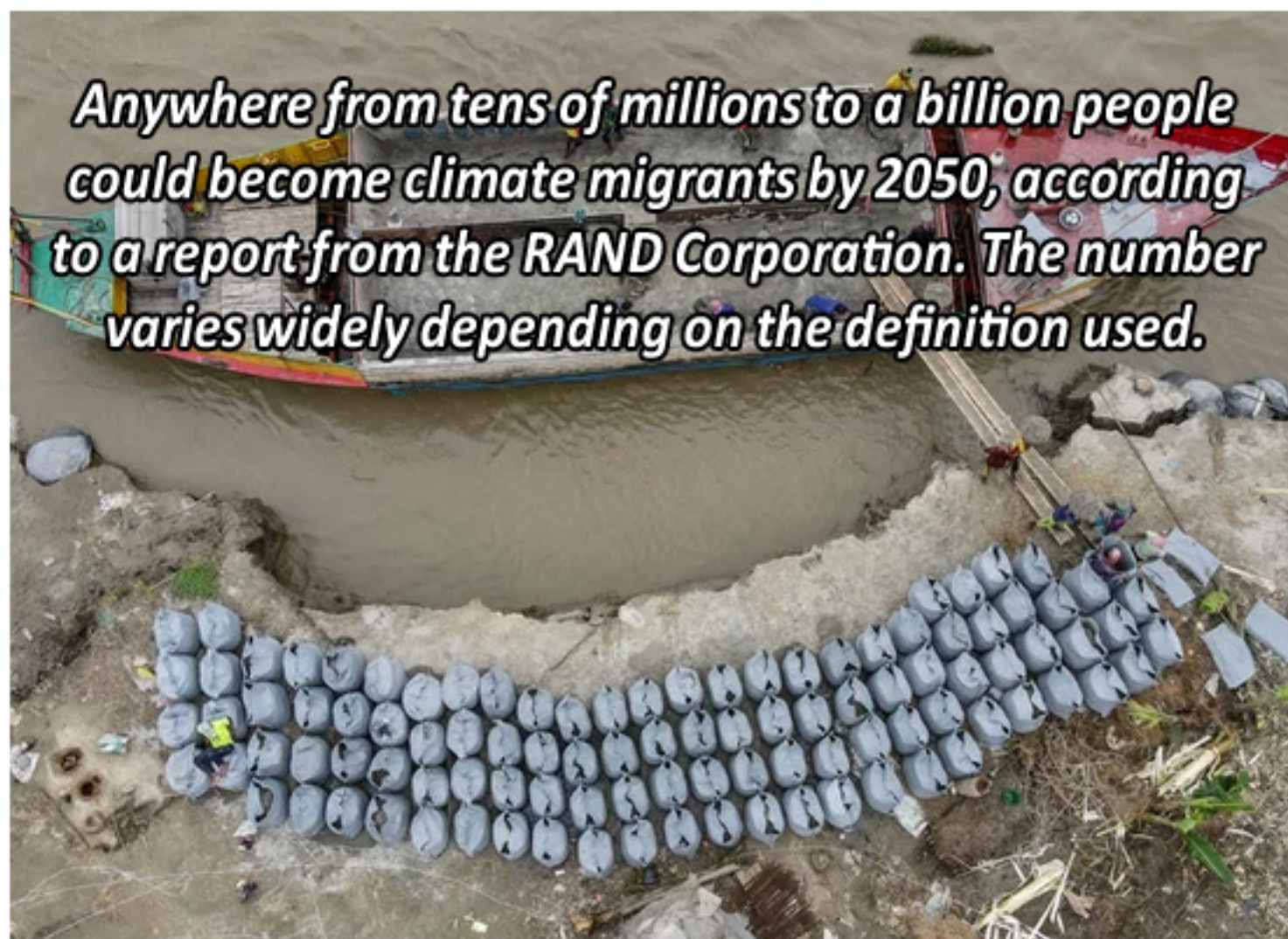
Workers place geo-textile bags to prevent river erosion on the banks of Padma River in Bangladesh
